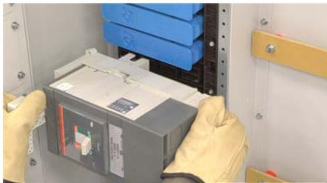
The Breaker Is Inserted Into The SafePanel
